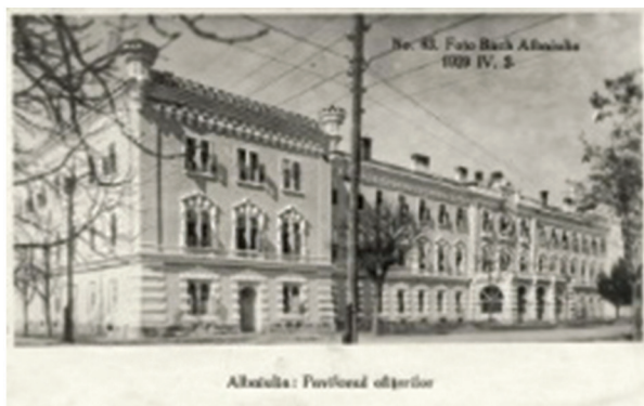
38. THE OLD BUILDING, HOSTING OFFICERS
