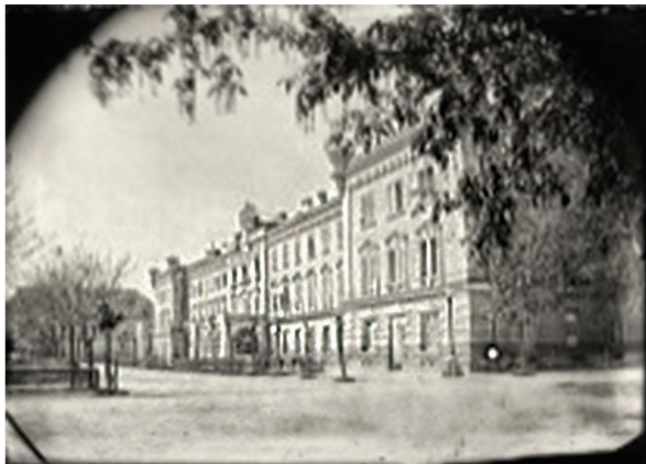
37. THE OLD BUILDING, HOSTING OFFICERS
